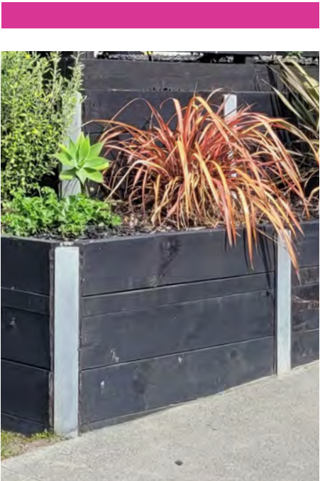
TIMBER / STEEL BEAM RETAINING WALL
